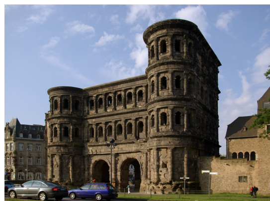
Fig. 10 Trier (Germany), the exterior side of the Porta Nigra.
